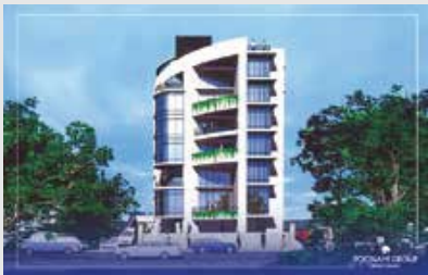
Poonam's Building Juhu, Mumbai
